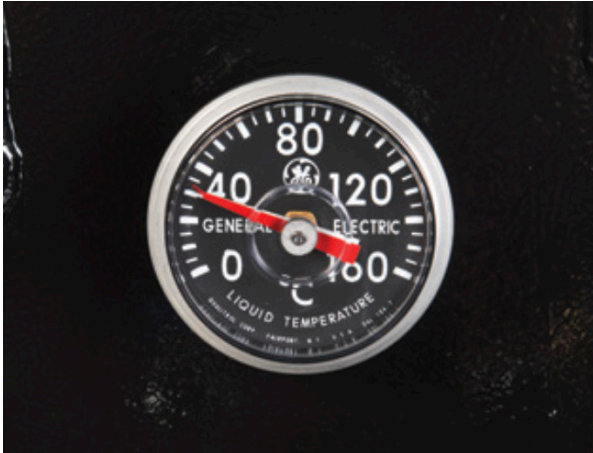
Main tank thermometer
