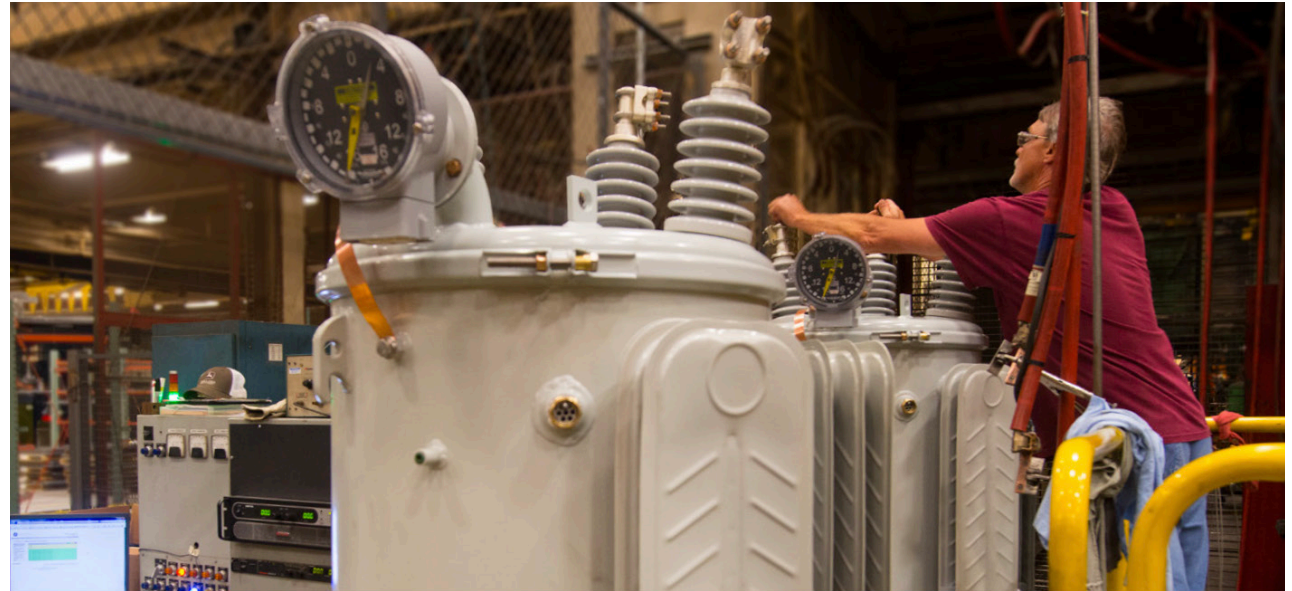
Complete electrical testing
