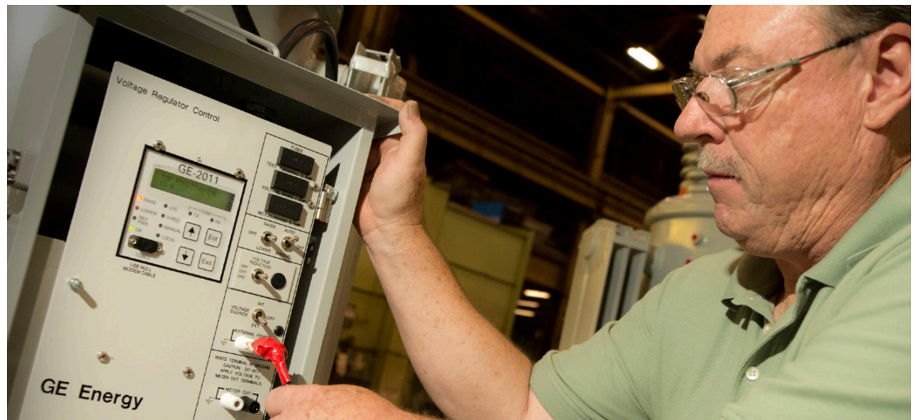
Controls programming and testing
